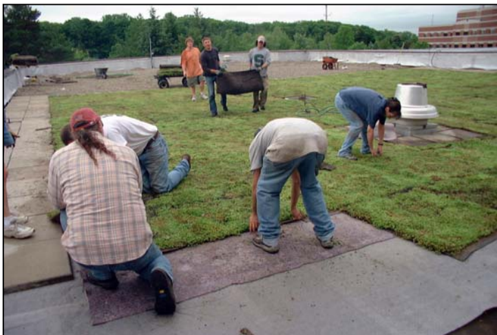
Installation of sedum 'sod' on roof of PSSB in May 2004
